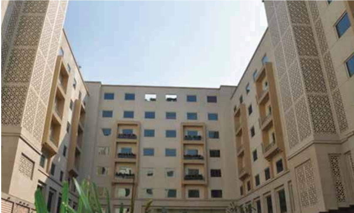
GRC Screens at Lemon Tree Hotel
