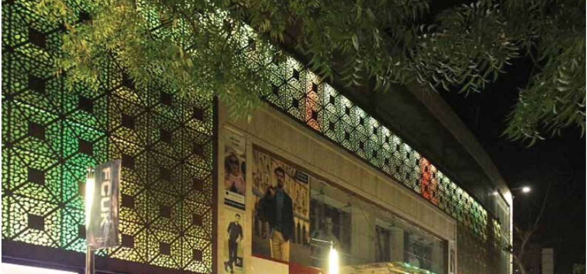
CNC Cut WeatherTex Board on Building Facades
